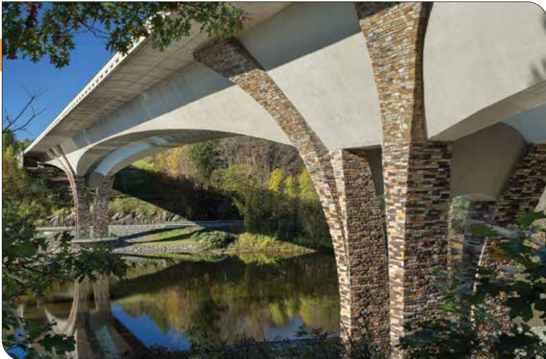
I-91 Brattleboro Bridge, Vermont, USA
